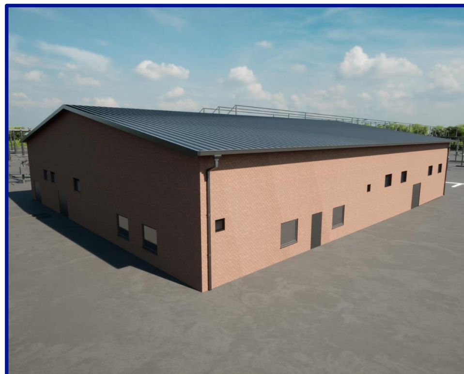
Figure 36: Monk Fryston Control Building Finish - Red Brick
