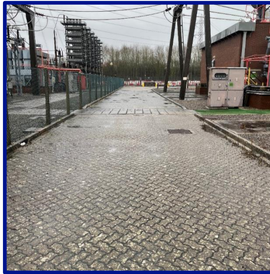
Figure 32: Block Paving (Source: MM Site Visit)
