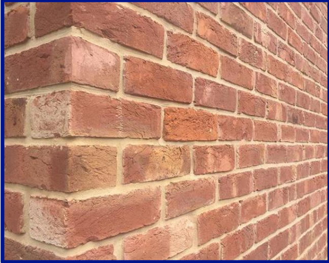
Figure 21: Red Brick (Source: Ammaari Stones)
