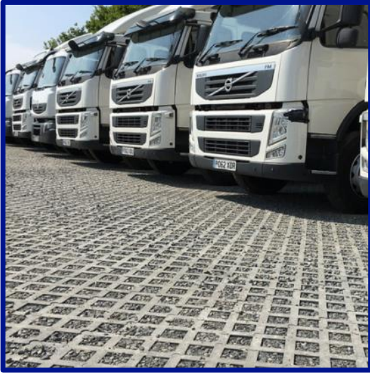
Figure 29: Truck Grid (Source: GrassMats Ltd)
