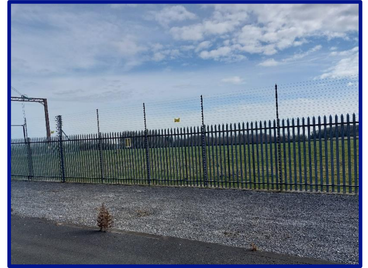
Figure 30: Security Fence (Source: MMD Site Visit)
