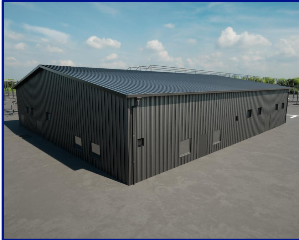
Figure 37: Monk Fryston Control Building Finish - Grey Cladding
