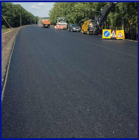
Figure 31: Impermeable Tarmac Road (Source: Swift surfacing)
